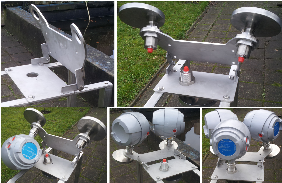
Figure 1.7: Installation sequence of the standard Point Array mounting frame for the WaveGuide Direction radars.
