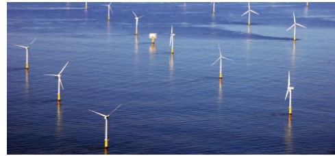
Figure 4: Aerial view of Princes Amalia Wind Park.
